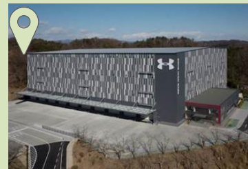
Construction of a Large distribution warehouse with seismic isolation structures (Iwaki City , Fukushima)
