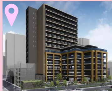
Utilization of former company dormitories for Financial Institution (Nagoya City , Aichi)
