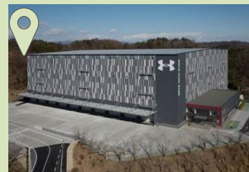
Construction of a Large distribution warehouse with seismic isolation structures (Iwaki City , Fukushima)
