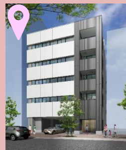
First construction work order received in the Chugoku area (Hiroshima City , Hiroshima)
